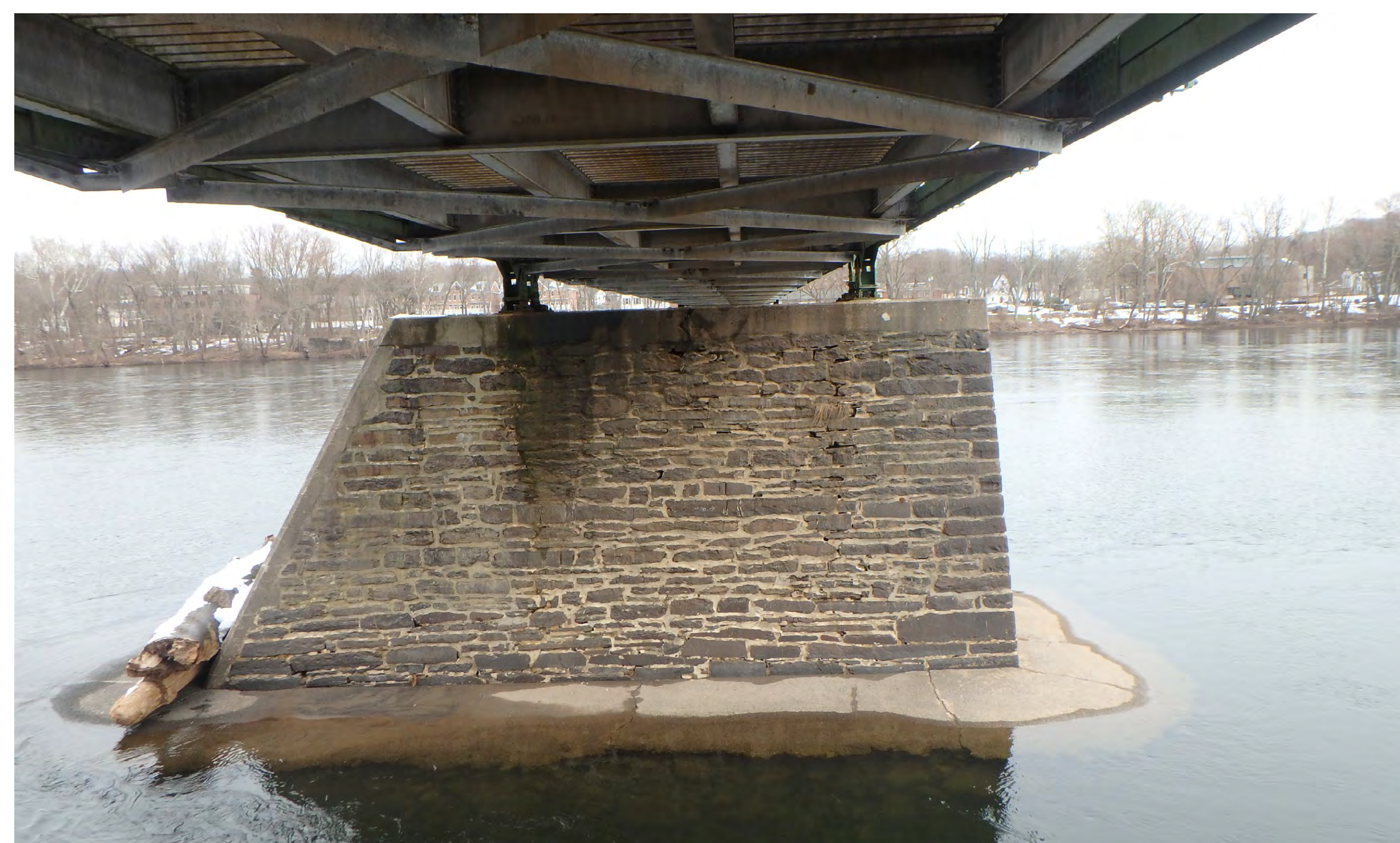
Missing Mortar
