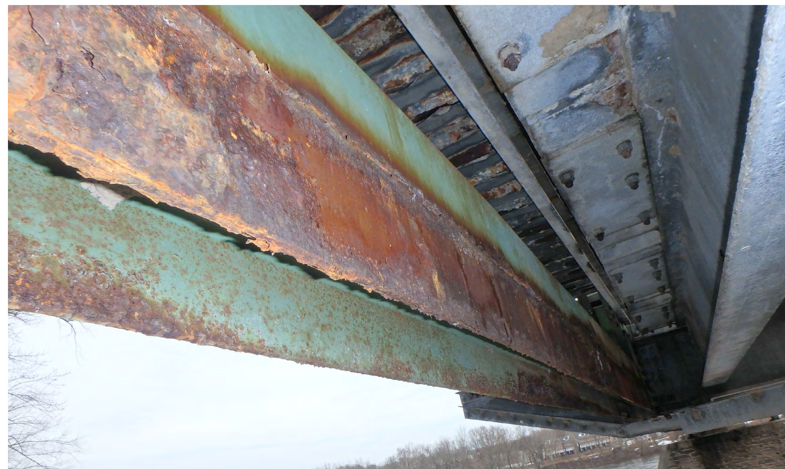
Paint Deterioration
